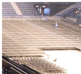
Low Row Rise System - An alternative option where height is restricted. Seats have to be completely removed before retraction.
