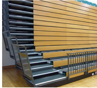
Self-storing Side Rails - Angled to nest together when unit is retracted.
