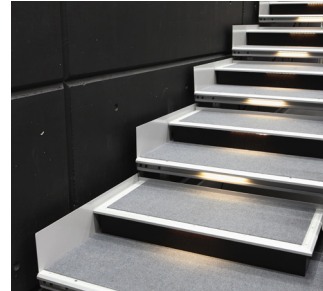
Kick plates - To guard the operational clearance where an aisle is adjacent to a wall.
