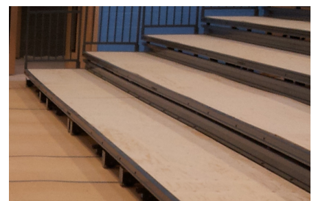
3/4" plywood deckboards (for finishes, see page 4).
