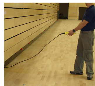
Type V - Travelling unit which allows movement as a complete bank, forwards and backwards, from its stored position.
