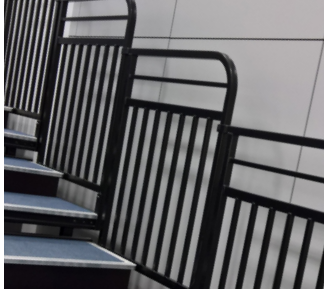
Type D - Tubular steel infill.
