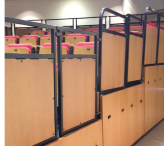
Type B - MDF infill, faced with melamine (finish: oak) - other finishes on request.
