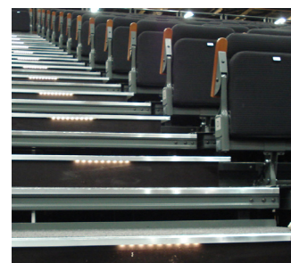
Aisle Lights - Low voltage, low glare, LED lighting with optional one hour battery back-up and dimming function.
