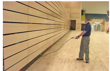
Type V - Travelling unit which allows movement as a complete bank, forwards and backwards, from its stored position.
