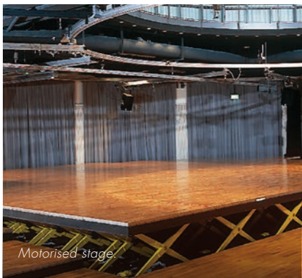
(This photo and photo above) Airstage used as variable height floor at University of Sussex, UK.
